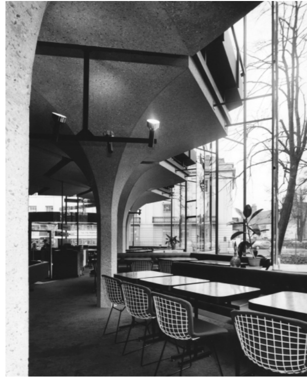
Patrick Gwynne's foyer at York Theatre Royal, seen in 1968, showing the hexagonal concrete columns
